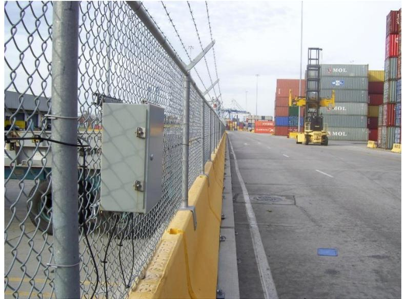
Southwest Microwave's MicroPoint™ Cable system pinpoints fence cut or climb attempt to within 3m, while ignoring environmental disturbances such as wind, rain or vehicle traffic.
